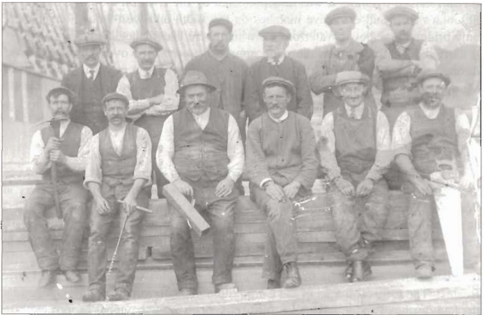
Repairs to Cox's Bridge Foreman Laurence Farrell with beard and cap
